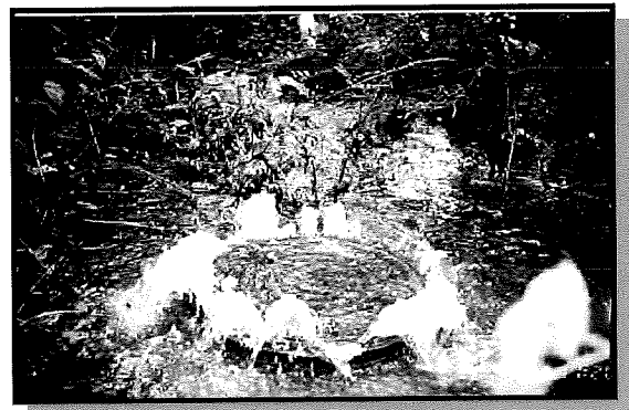
SSOs include untreated discharges from sanitary sewer systems that reach waters of the United States (photo: US EPA).
