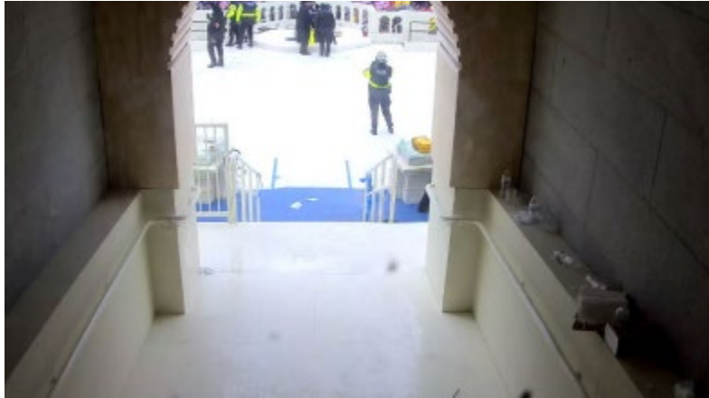
Image 2 (The “Tunnel” as seen on CCTV footage prior to rioters entering)
