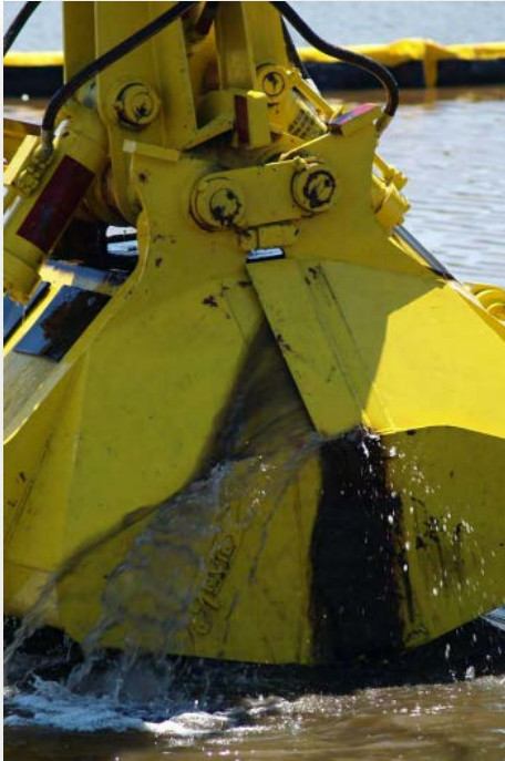
Dredging at Stryker Bay. Photo credit: MNDNR.
