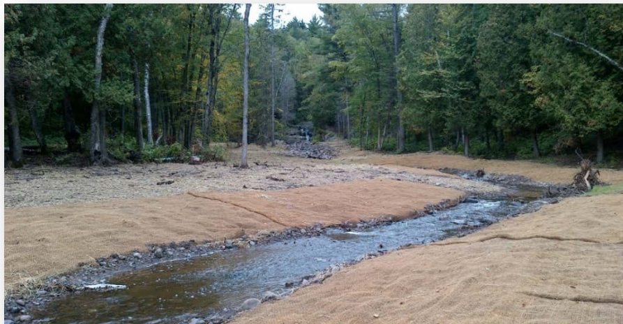
Restoration at Knowlton Creek. Photo credit: MNDNR.
