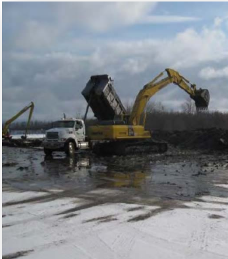
Tallas Island winter mechanical excavation. Photo credit: MPCA.
