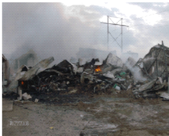
Warehouse after fire
