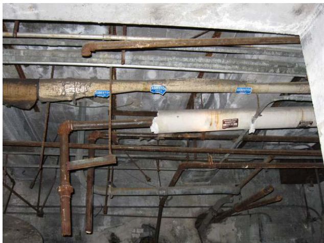
Asbestos-labeled pipes
