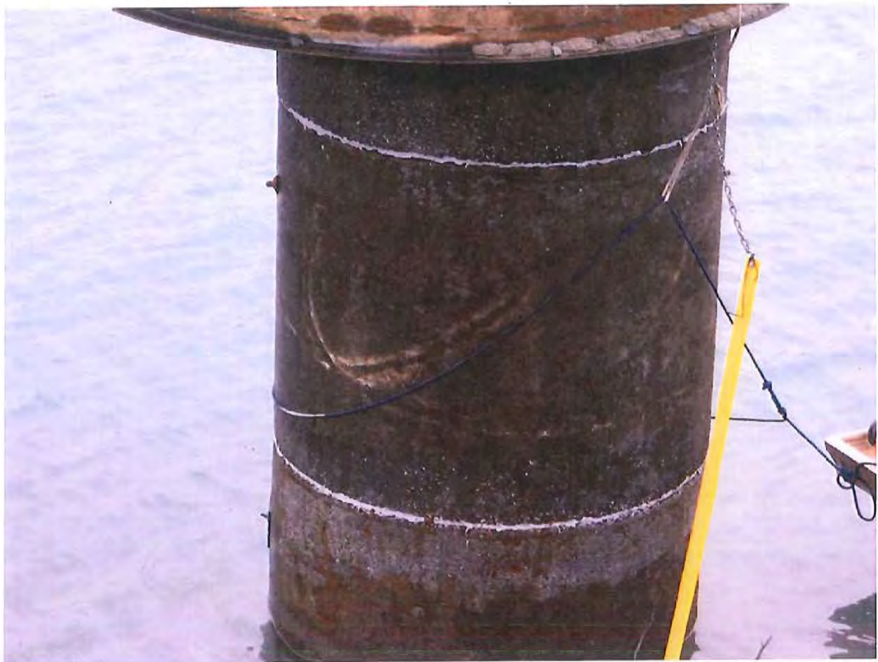
Photograph 14. 3/19/14 photograph of new grout on CAPE FEAR coal ash basin riser.
