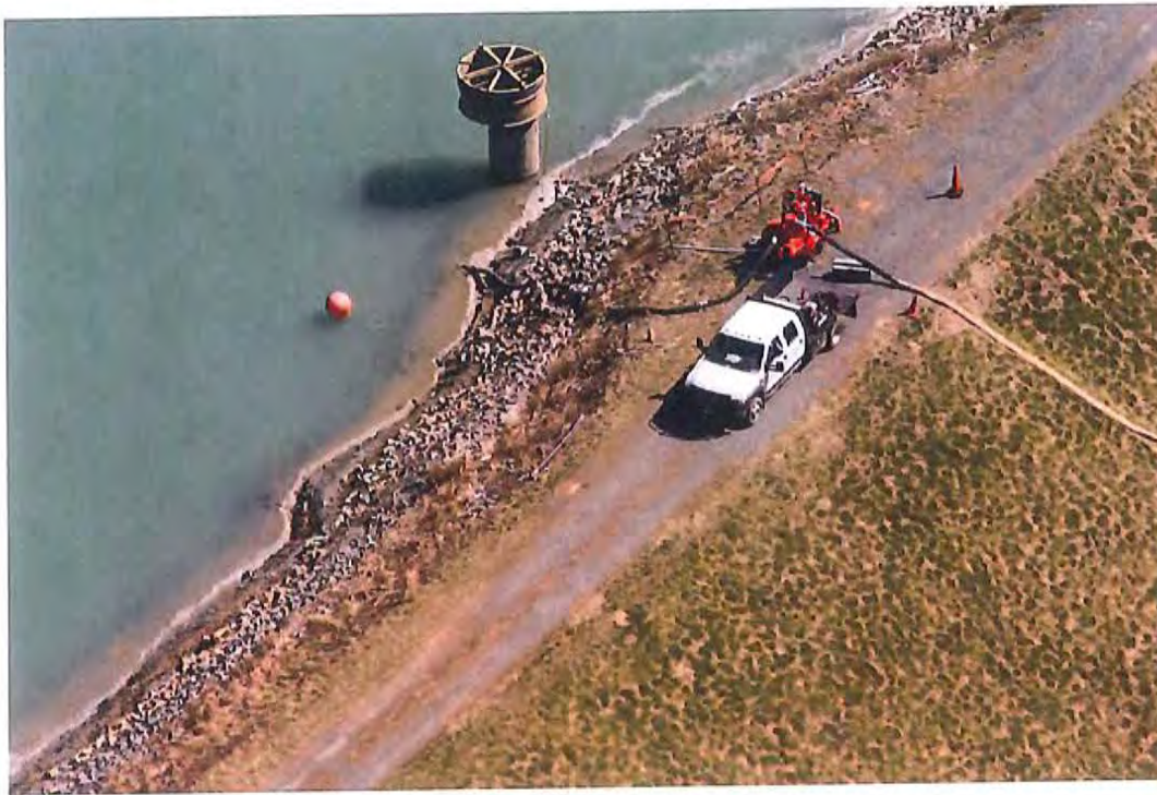
Photograph 10. 3/11/14 aerial photograph of CAPE FEAR 1985 coal ash basin with Godwin pump and truck.
