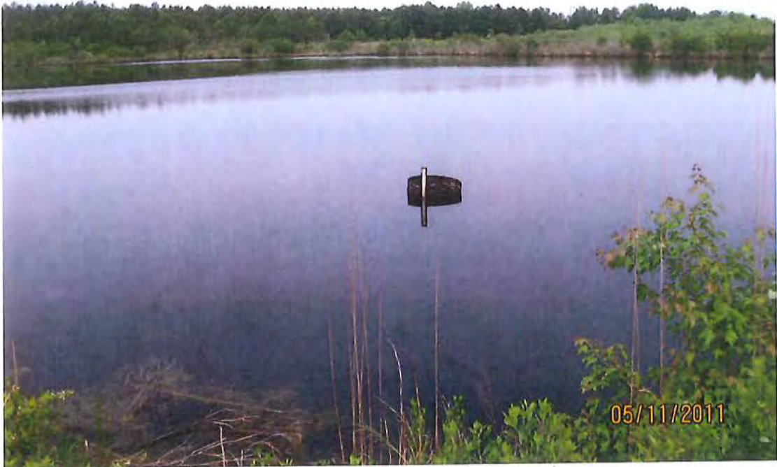
Photograph 5. Riser in CAPE FEAR 1978 coal ash basin from 2012 Five Year Independent Consultant Report.
