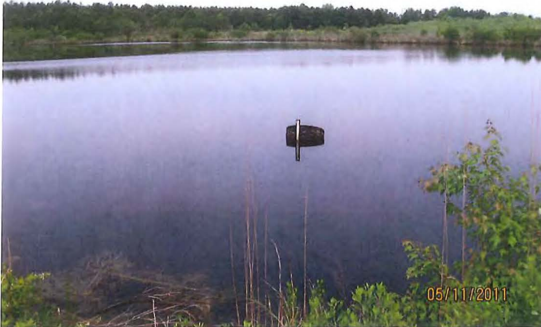
Photograph 5. Riser in CAPE FEAR 1978 coal ash basin from 2012 Five Year Independent Consultant Report.
