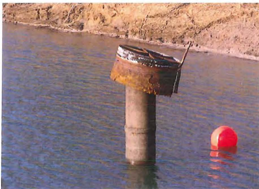
Photograph 11. 3/19/14 photograph of CAPE FEAR 1978 coal ash basin riser, prior to repair work.
