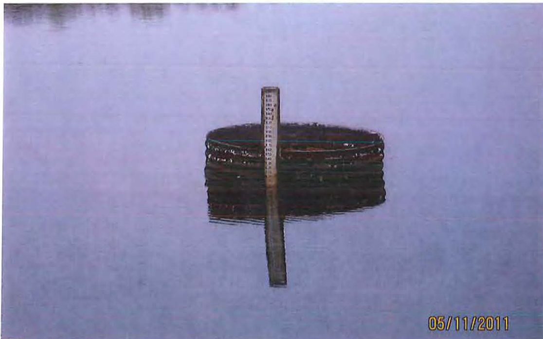
Photograph 6. Riser in CAPE FEAR 1978 coal ash basin from 2012 Five Year Independent Consultant Report.
