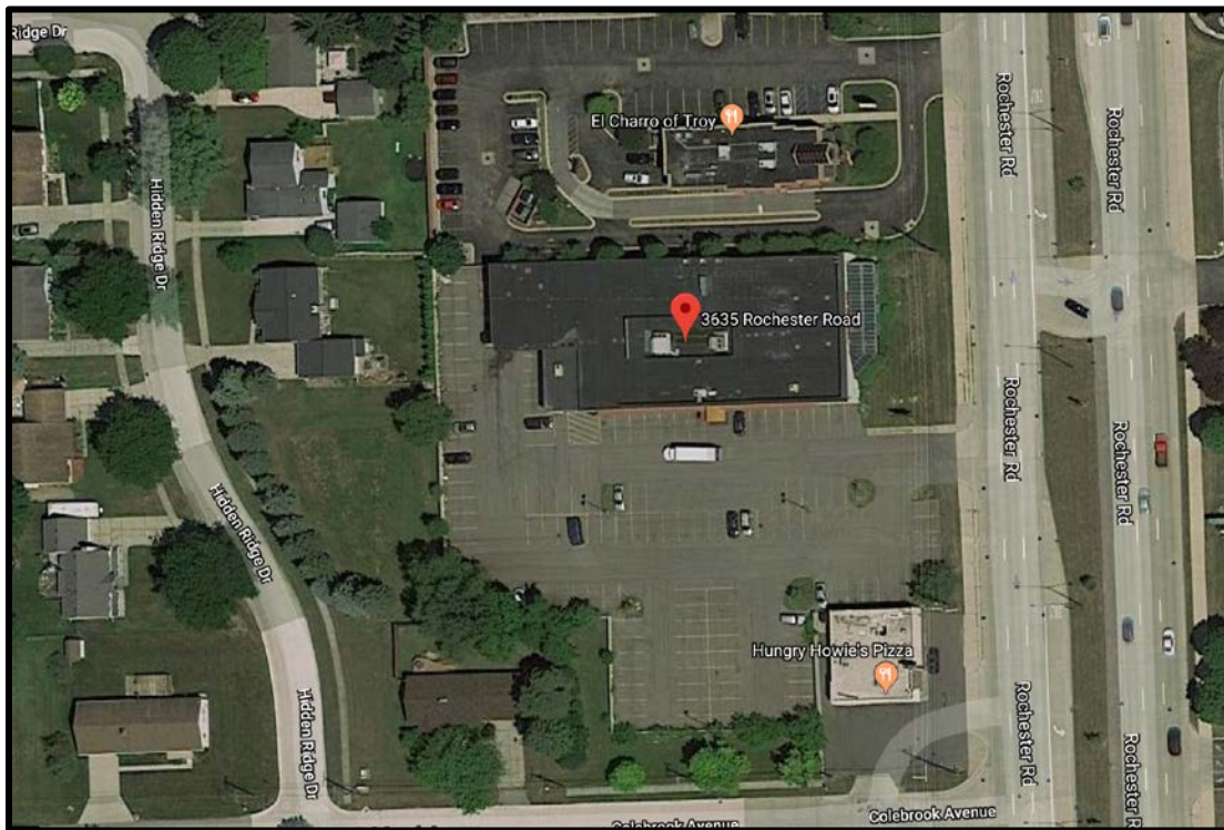
Picture 1: Satellite Image of the Subject Property at 3635 Rochester Road
