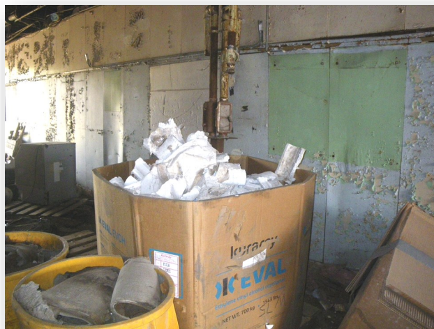
Illegally removed asbestos pipe insulation
