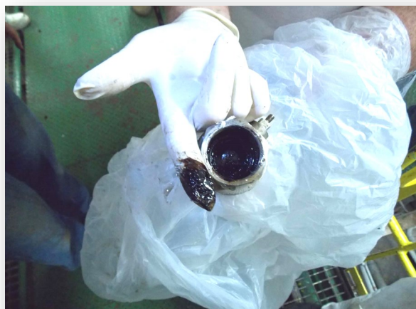
Oily by-pass pipe
