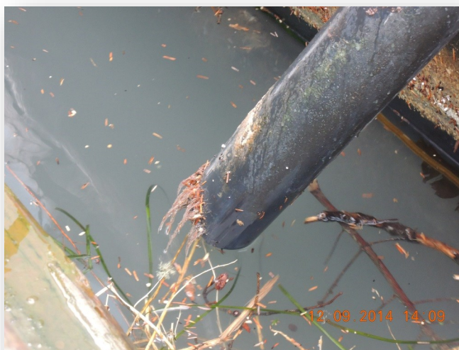
Pipe directly discharging overboard from restroom
