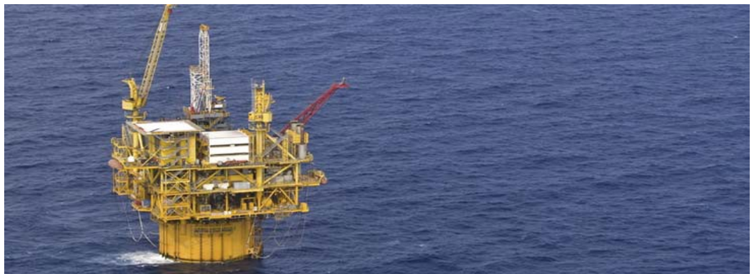
Outer Continental Shelf Oil Rig, Bureau of Ocean Energy Management
