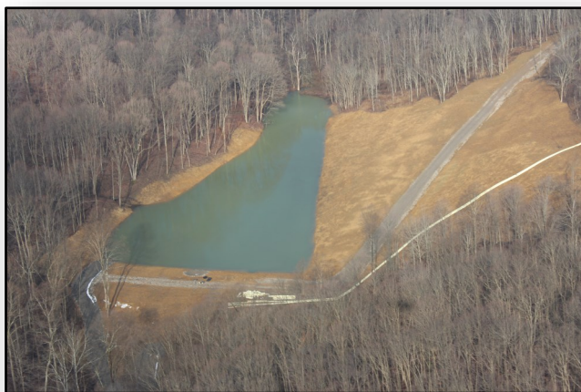
Aerial view of illegal impoundment
