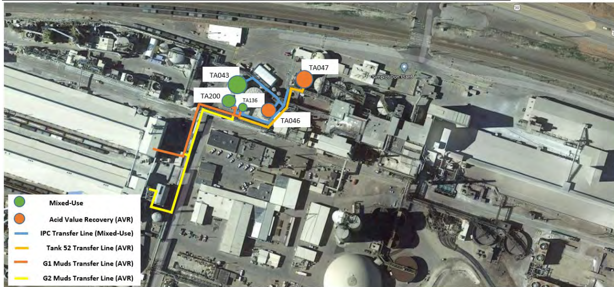
Figure 8: Muds & 52% Acid Transfer from Phosphoric Acid Plant to Granulation 15
