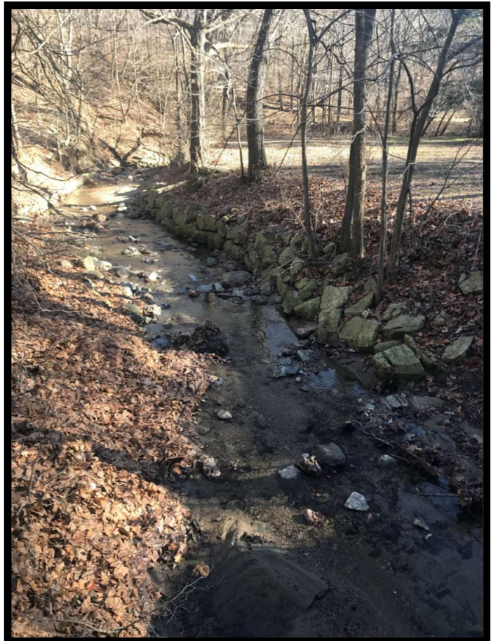
Looking Downstream of downstream extent at Turkey Creek below Black Bridge
