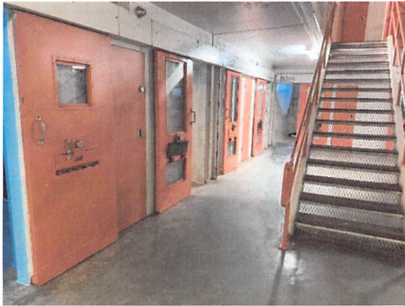
Prior to repainting
