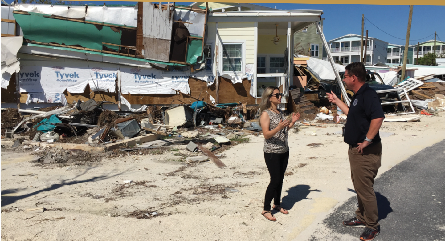
▲ Natalia Casella, CRS Program Specialist, and Tim Haugh, U.S. Citizenship and Immigration Services Supervisory Community Relations Officer – Southeast Region, survey damage from Hurricane Irma in South Florida. They both served as volunteers with FEMA's Surge Capacity Force (SCF) interagency effort. (U.S. Department of Justice)
